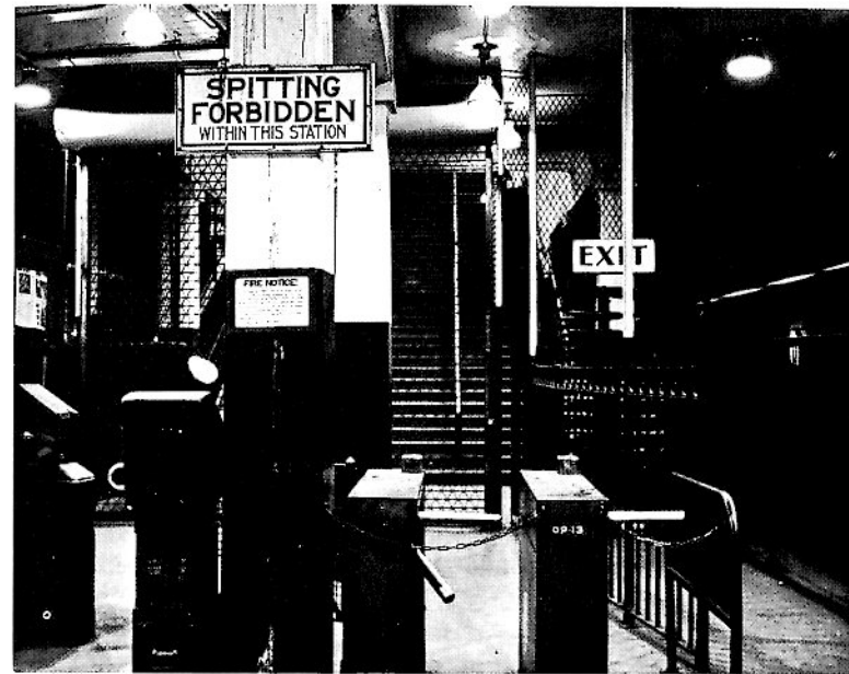
FIG. 29. The nether world of the subway
